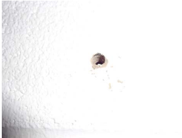
PHOTO 1 – SOUTHWEST CORNER BLOCK WALL Empty Cavity
