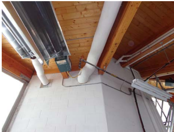
PHOTO 2 – CEILING T & G WOODEN STRUCTURE
