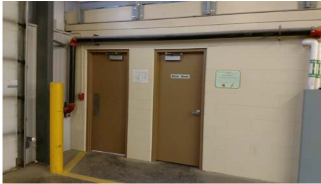
PHOTO 1 – Cindercrete Block Wall
